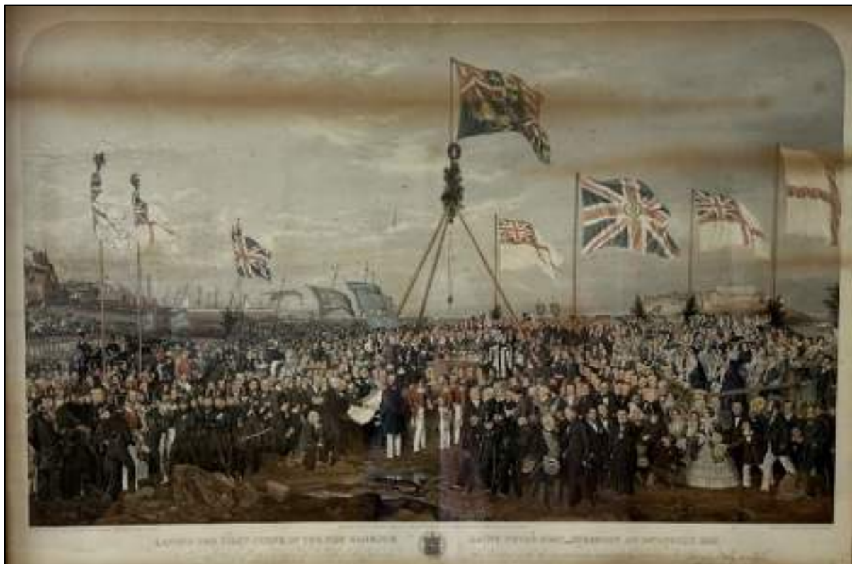
Image of the laying of the first stone at St Peter Port Harbour 24 th August 1853, displayed in the Royal Court.
