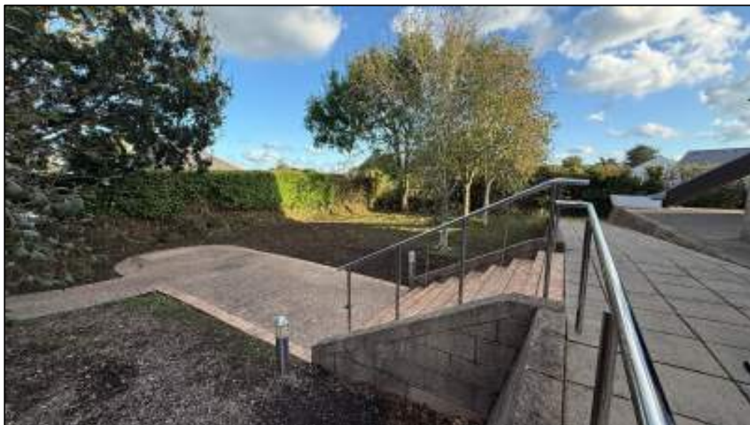
Works carried out during 2025 to landscape the garden with new hedging and plants
