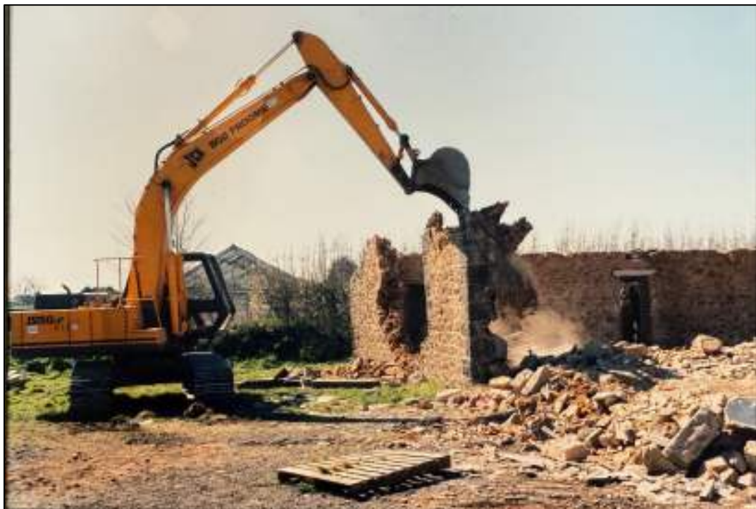
Demolition of Dauntless Hall
