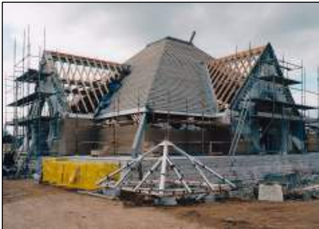
Construction of the Pyramid feature of the Masonic Centre this enabled the building to remain the same size as the Dauntless Hall structure
